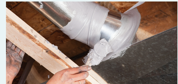
Duct sealing
